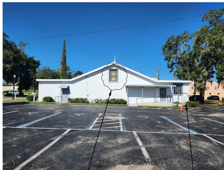
STAINED GLASS TO BE REMOVED & PRESERVED
